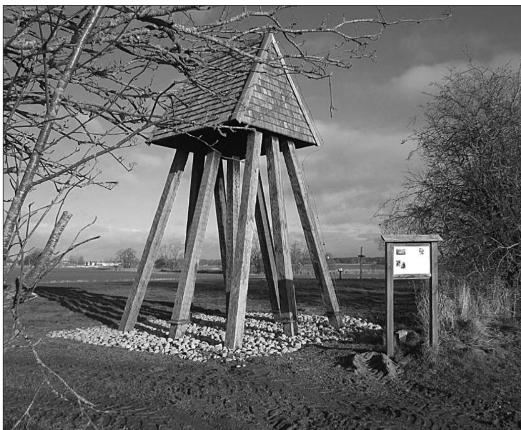
24 tons hand-laid kullersten, now together with the drainage, offers the possibility of air circulation around the legs. Foto Truls Wiberg
